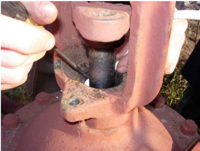
Picture 1 Repair of valves
